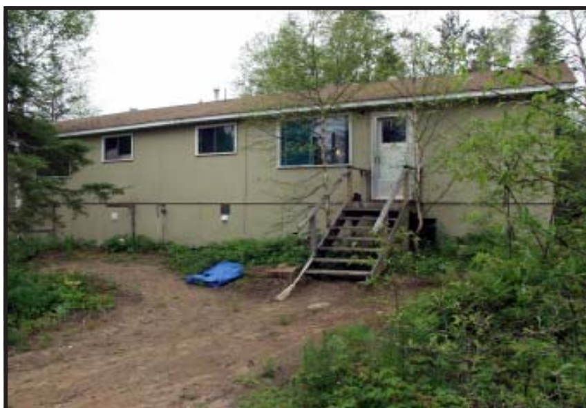
This four-section, eight-bedroom complex, constructed in 1972, is one of the residential buildings scheduled for replacement within the next year.
